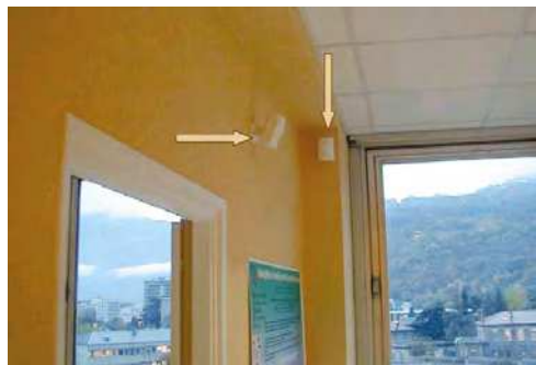
Fig. 2. Infrared (arrows) for localizing dependent people in a health smart home
