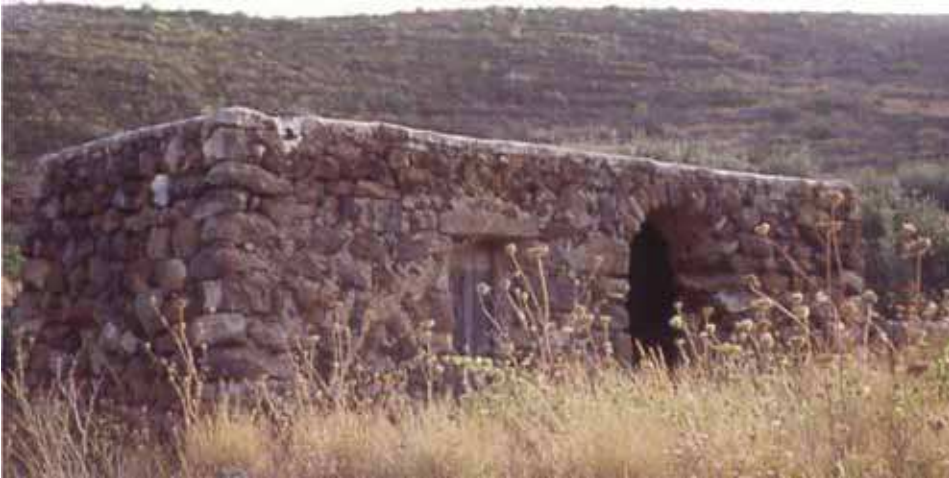
Figs. 13 - 14. Traditional building typologies. The use of appropriate materials, the bioclimatic relationship with the context contribute to maintain a constant internal microclimate without integration systems. "Dammusi" of Pantelleria and Apulian "trulli" are known as references in hot climates: the light painting favours the reflection of solar incident radiation.
