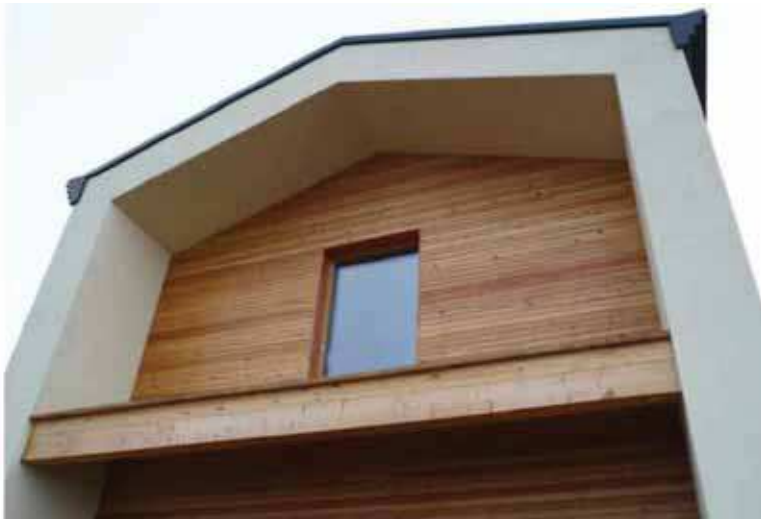
Fig. 5. Passive residential building in Montiano (FC - Italy), designed by Oficina 4, arch. G. Borghetti. The regular and compact shape helps the energy control; the orientation and limited size of transparent surfaces limit summer overheating.
