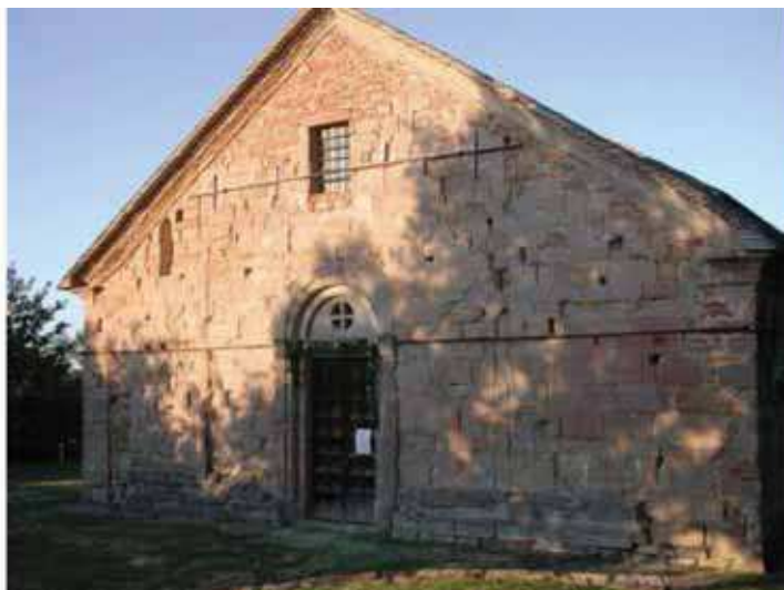
Fig. 2. Historical building. The Italian traditional architecture is characterised by envelopes built with considerable mass materials.
