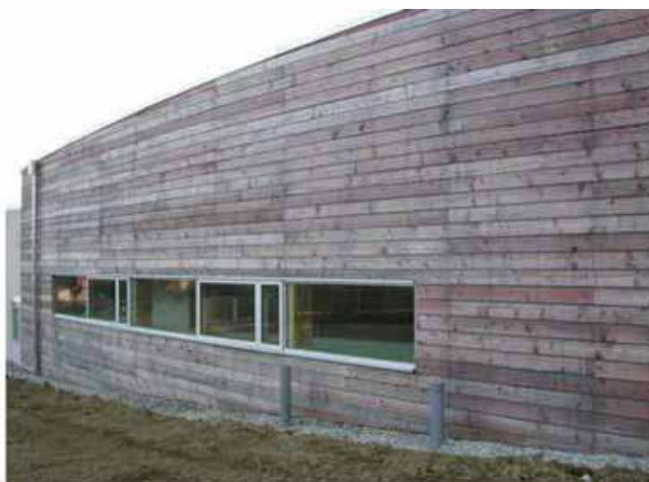
Figs. 8 - 9. The design of the School of Children in Ponticelli (Imola - Italy), arch. A. Contavalli, is characterised by energy efficiency. The north facade is extremely compact, the south one is glazed and protected by a system of external shields.
