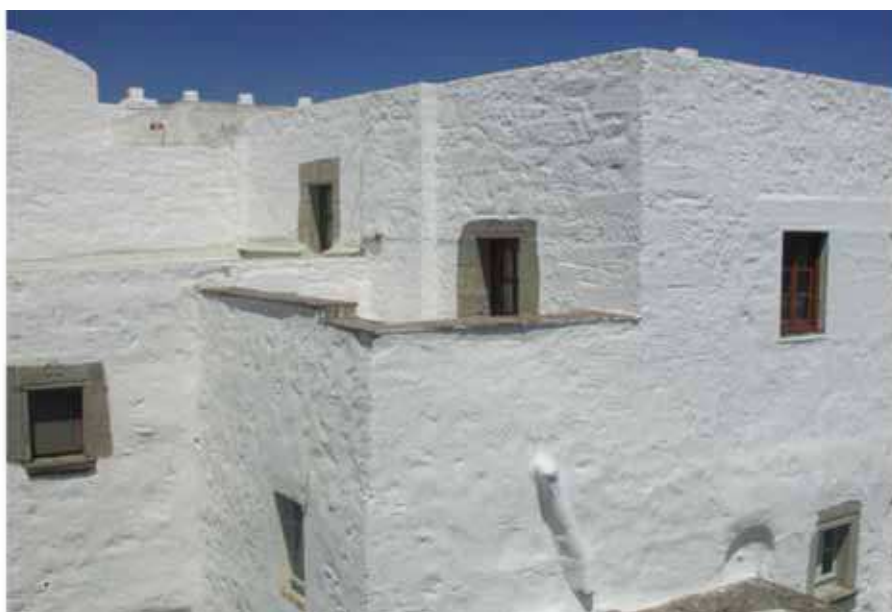
Fig. 15. Architecture and climate. The relationship with the climate and building traditions, often linked to local material availability, connotes typical construction
