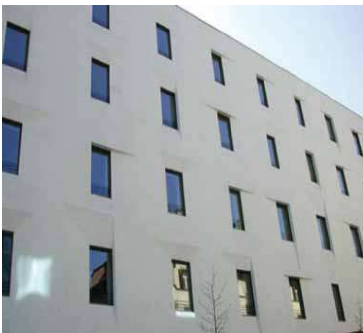
Fig. 4. Energy retrofit of the new headquarters of the Autonomous Province of Bolzano, arch. M. Tribus. This is the first national public building with a consumption of only 12 kWh/m 2 year for heating. It reaches the European standard of passive house. There is an outer coat of sintered polystyrene insulation 35-cm thick.
