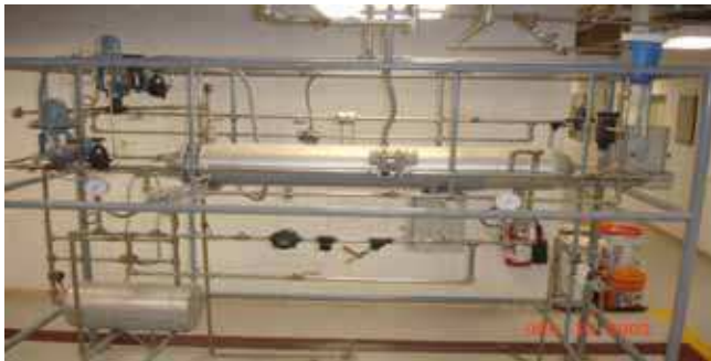
Fig. 17. Industrial heat exchanger used in the experiments.
