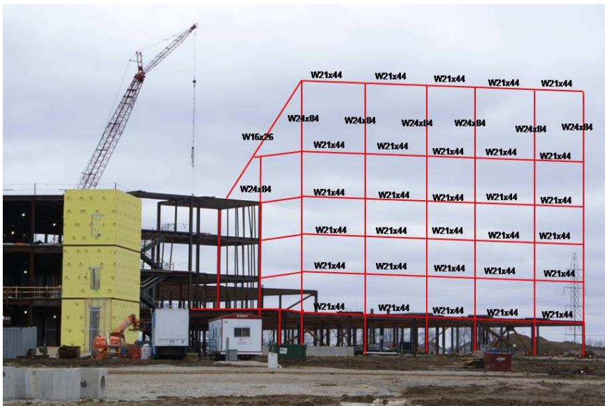
Fig. 9. A conceptual image of AR overlay of 3D design and contextual data (Dunston & Shin, 2009).
