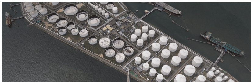
Figure 2. Typical onshore tank farm facility [2].
