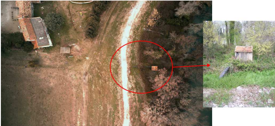
Fig. 6. 0.02 m resolution digital image acquired during the LiDAR survey. It shows a pump line through the base of a dike (source Cemagref -FUGRO)
