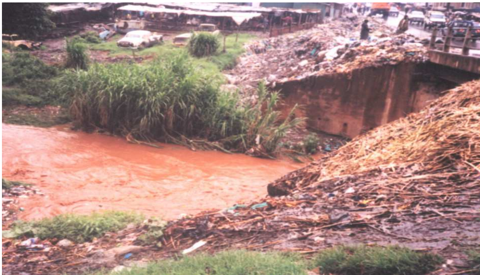
Photo 1. Gikomba-Shauri Moyo Bridge D/S Gikomba open-air market-solid wastes, Car shells and Jua Kali garages in the foreground.
