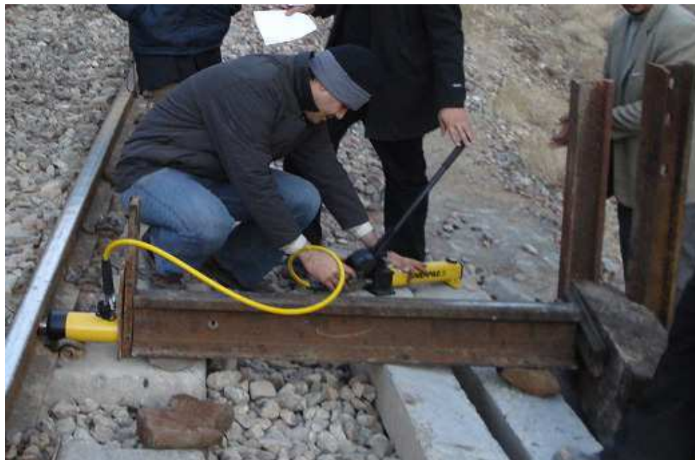
Fig. 15. Installation of the hydraulic jack
