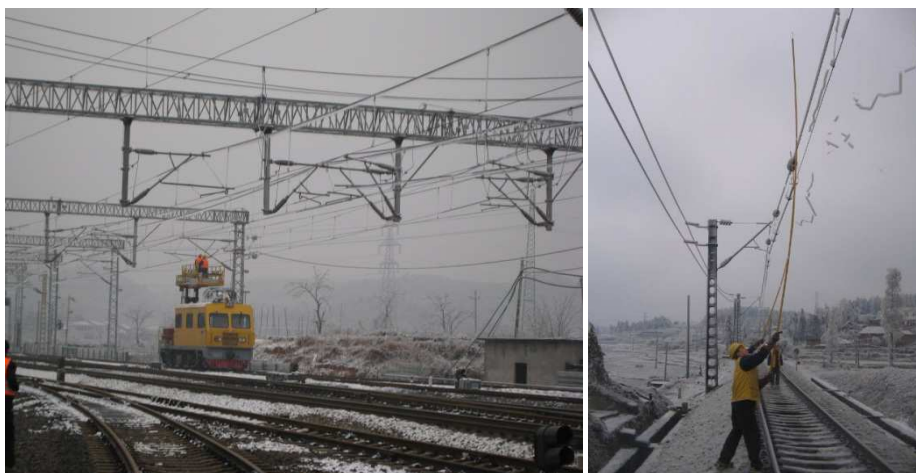
Fig. 1-1. Manual de-icing on overhead contact wires
