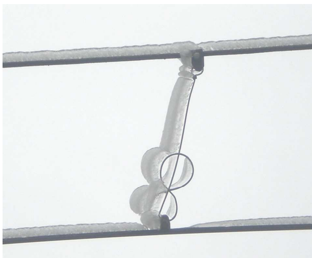
Fig. 2-2. Icing of contact wire
