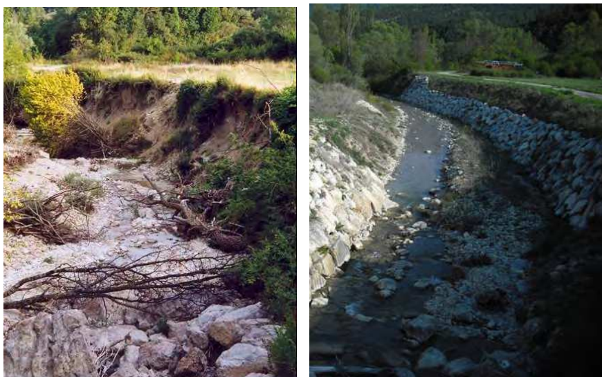
Fig. 9. The Céans river bed in 2004 (left) and in 2011 (right) (Southern French Alps). The bed of the Céans was entrenching strongly in the last decades, due to a great decrease of erosion and sediment transport. The river banks were falling regularly in the entrenched bed (left), obliging the authorities in building new embankments to protect surrounding areas from destruction (right).
