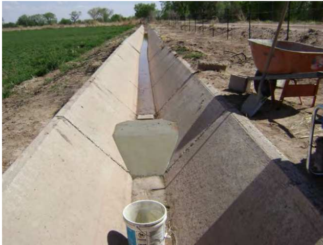
Fig. 5. Completed Broad Crested Weir for Field 3
