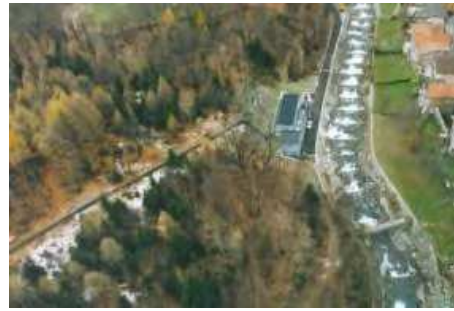
Photo 6. Rino: a view of the power station.
