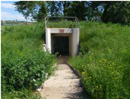
Photo 3. Armyary: the power house.
