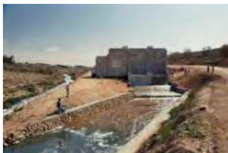
Photo 12. As Samra hydropower plant on the treated wastewater.
