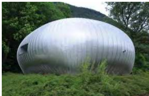
Photo 9. Seefeld: the power house.
