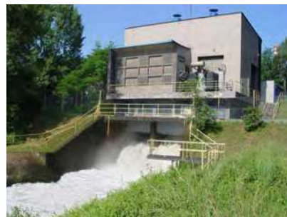
Photo 24. Skawina: the powerhouse during turbine overhaul.
