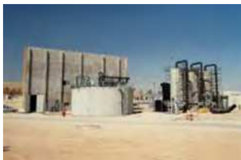
Photo 11. As Samra hydropower plant and wastewater treatment plant inlet structure.
