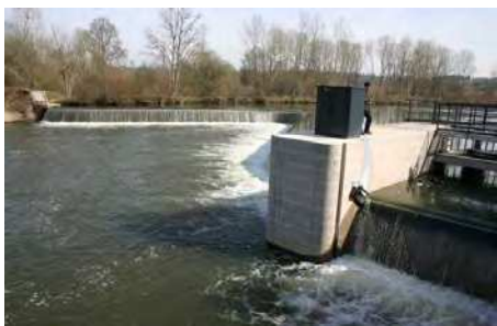
Photo 19. L'Ame: downstream global view of the dam and the turbine.
