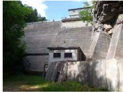
Photo 16. Le Day: The foot of the dam where the small power plant will be set.
