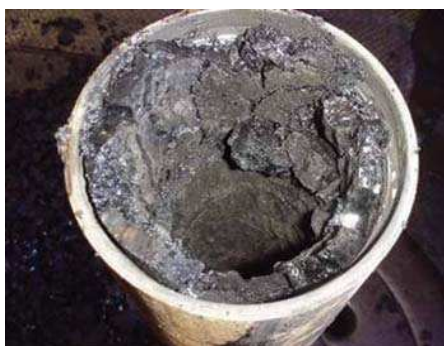
Fig. 1. Asphaltenes clogging a pipe. Courtesy of A. Pomerantz, Schlumberger.
