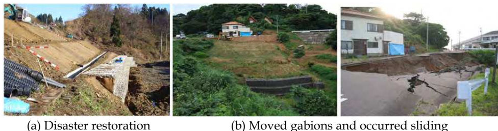
Photo 11. Application of large-scaled gabion at present
