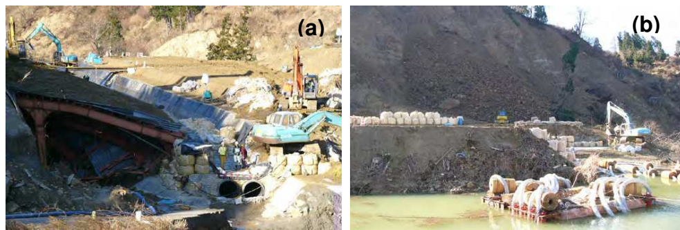
Fig. 4. Emergency works at Higashi Takezawa landslide dam. Photo taken on 20.12.2004 by Takeji & Tadashi, 2005
