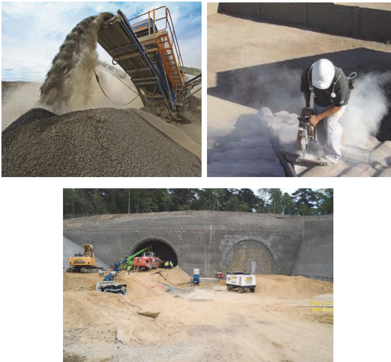
Fig. 1. Job processes that generate and disperse respirable silica dusts into the air
