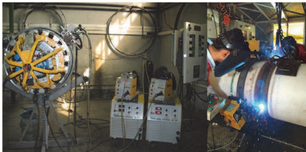
Fig. 5. Automatic pipe line welding system in the experiments (made by Novin Sazan Co.)
