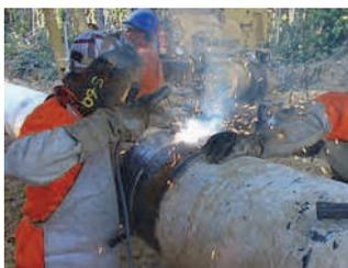
Fig. 30. Pipeline manual welding procedure.
