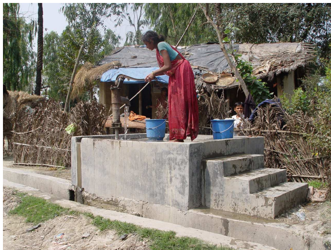
Fig. 5. Example of 'flood-proofed' water well (Photo: courtesy of Jørgen Kristensen, Danish Red Cross)
