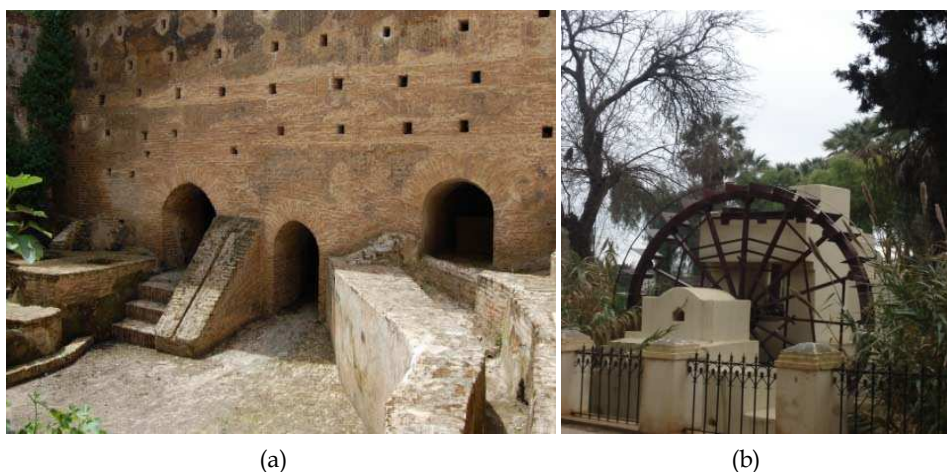
Fig. 5. a) Water distributor, Fes b) Noria from which the water flowed to the distributor
