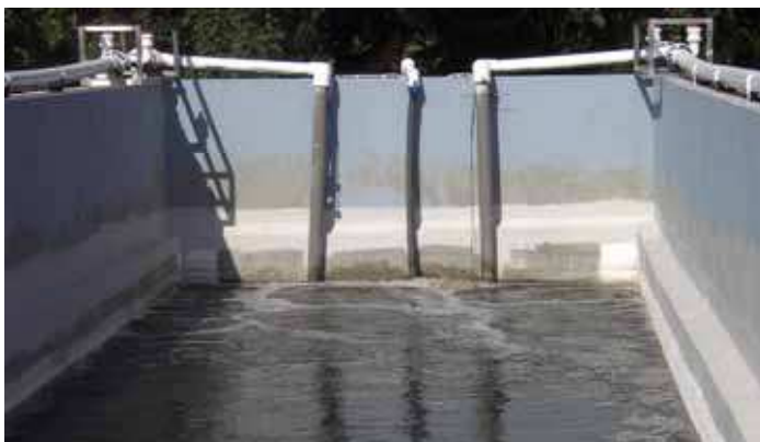
Fig. 13. Wastewater treatment system at Catapereiro
