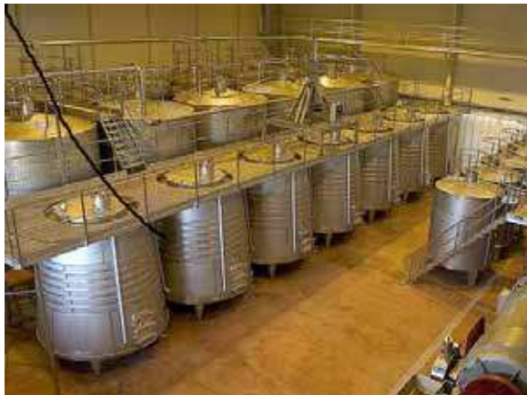
Fig. 10. Mingorra winery unit
