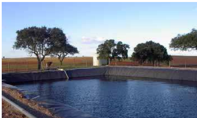
Fig. 14. Wastewater treatment system at Mingorra
