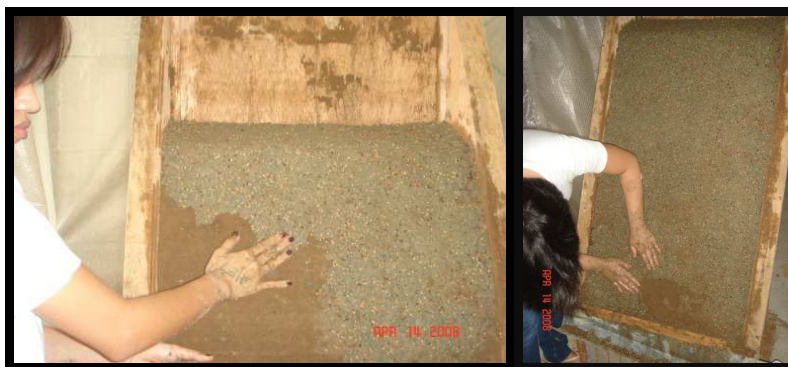
Fig. 4. Hydroseeding by manual application
