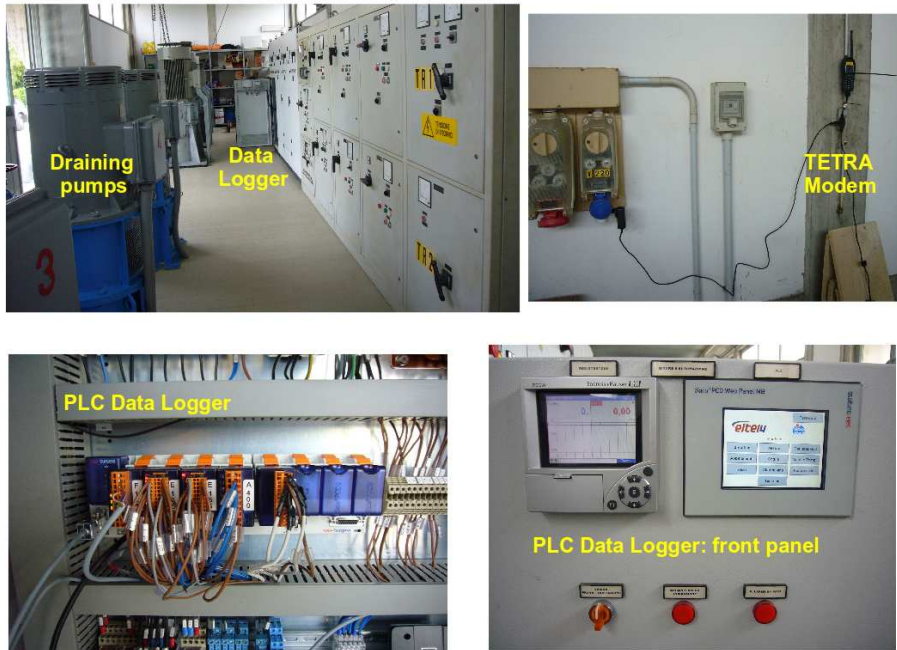
Fig. 9. Draining pump located at “Mordano” city.
