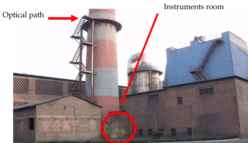
Fig. 17. Another testing place for in situ on-line monitoring of industrial emissions.
