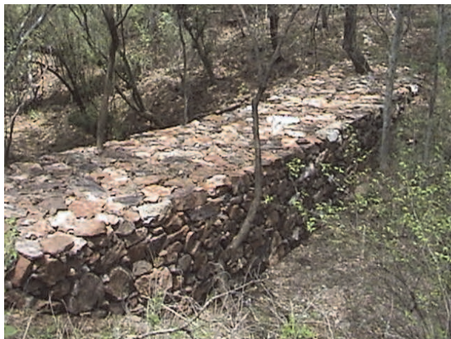
Fig. 3. Retenidas for runoff control in La Labor
