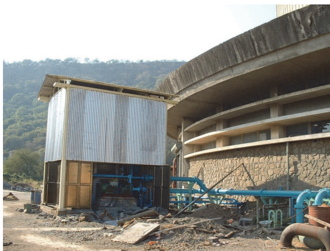
Fig. 4. Desalination unit located outside Cirus annulus area
