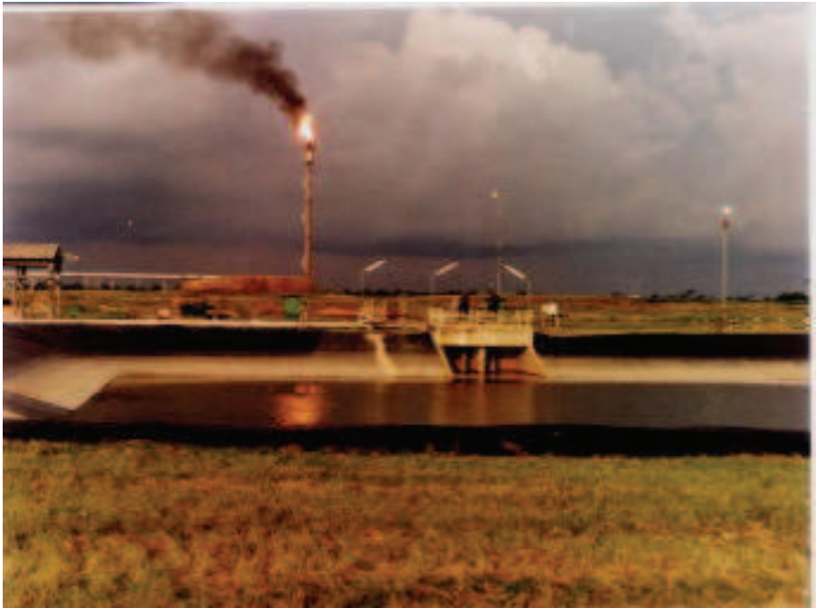
Plate 4. Emissions from a Petrochemical plant
