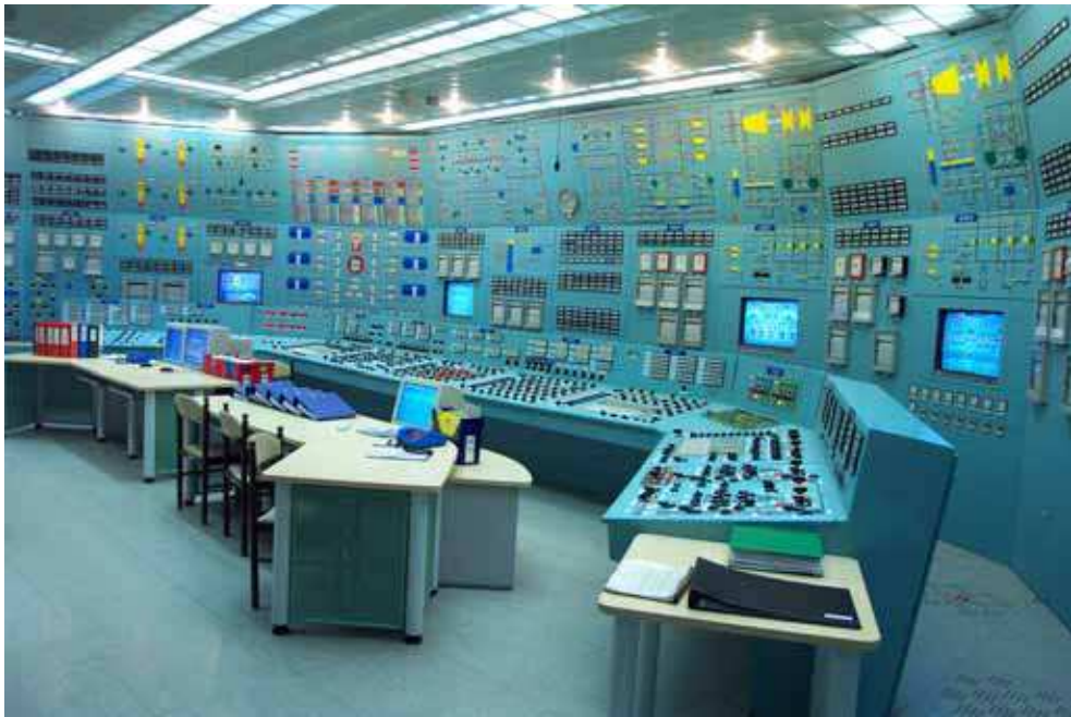
Fig. 3. The replica control room of the Paks NPPs training simulator
