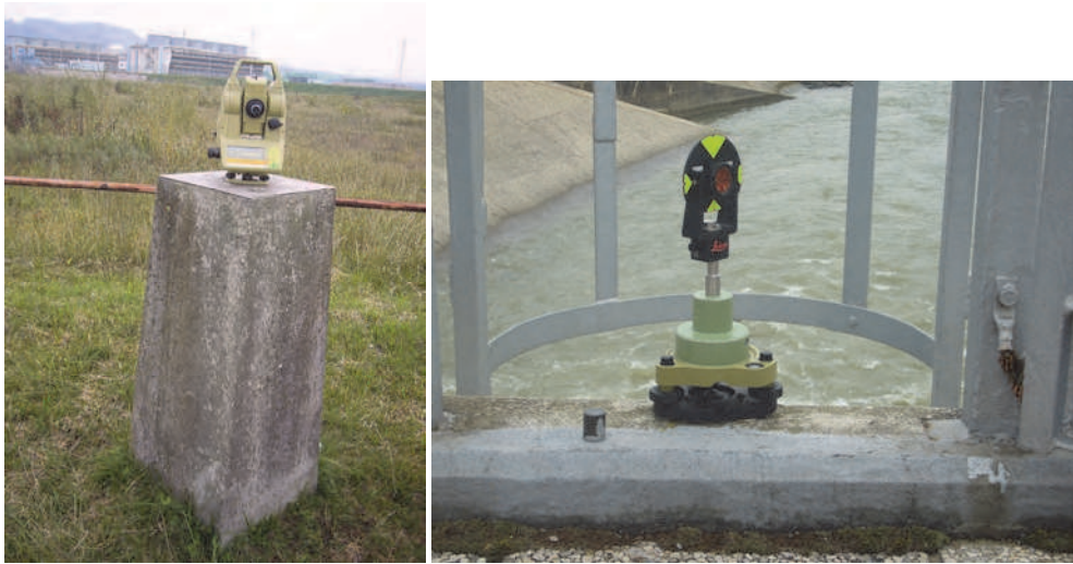
Fig. 1. Stabilisation and signalisation of the reference and control points
