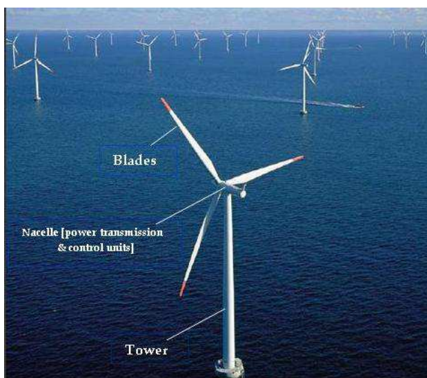
Fig. 1. Offshore horizontal-axis wind turbine
