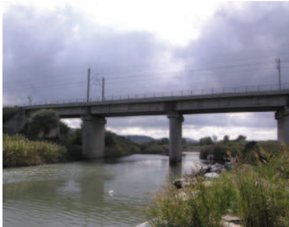
Fig. 1. Sinello railway bridge (Garibaldi et al., 2005).
