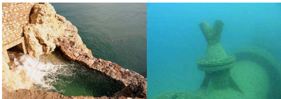
Fig. 3. Photographs of brine discharge configurations located in Spain. .A) Dicharge trough a submerged outfall. B) Surfice discharge .C) Discharge trough multiple jets (CEDEX).
