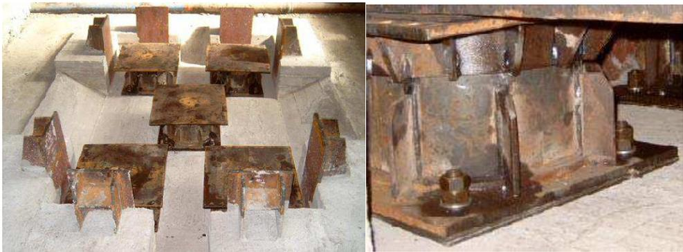
Fig. 2.16. Alternative 2 bolster for heavy equipment
