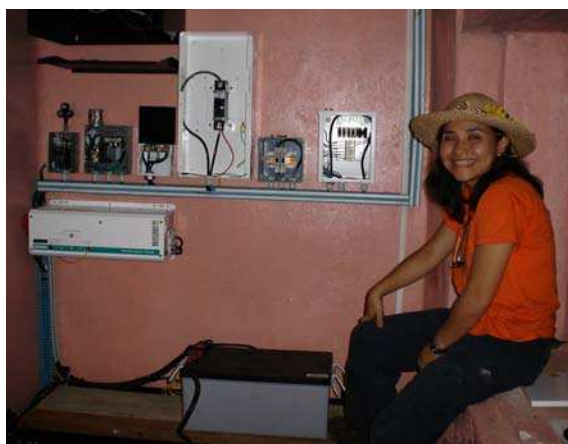
Fig. 13. COHCIT Sososal PV satellite telecenter with internet connectivity using quality BOS components with SOLARIS installer Ethel Enamorado in Lempira, Honduras.
