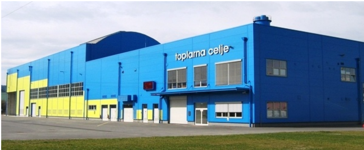
Figure 8. Celje W-t-E plant [3]
