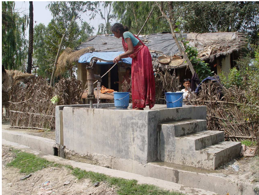
Fig. 5. Example of 'flood-proofed' water well (Photo: courtesy of Jørgen Kristensen, Danish Red Cross)
