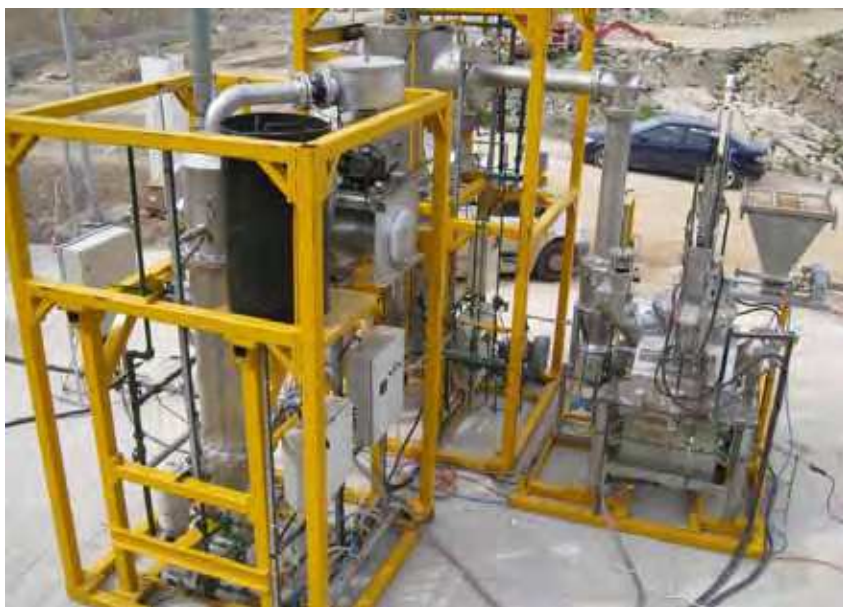
Photo 5. Another general view of the demonstration gasification / vitrification unit
