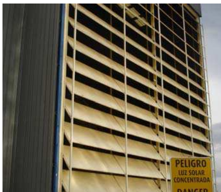
Fig. 10. Attenuator of the solar furnace of PSA (Almería Solar Plant)
