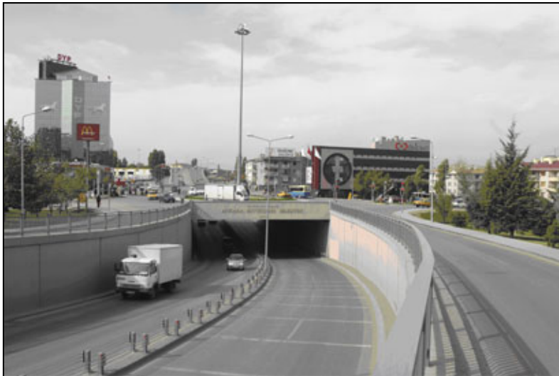
Figure 7. An underground road in Ankara [44].
