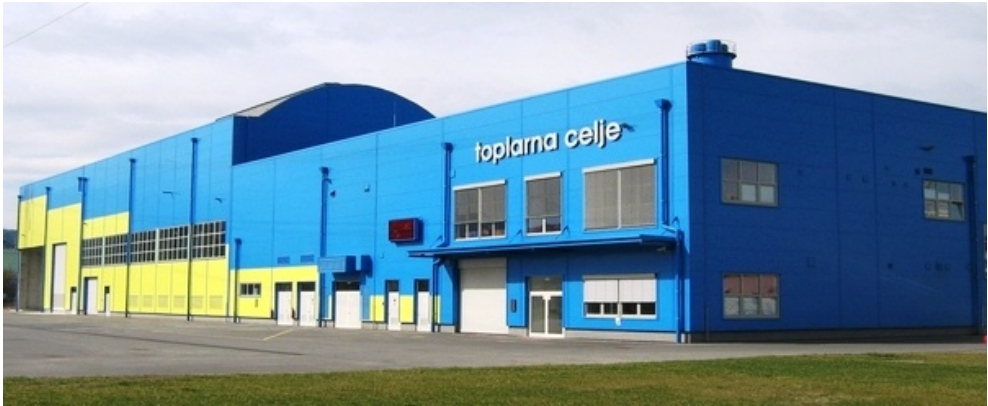
Figure 8. Celje W-t-E plant [3]
