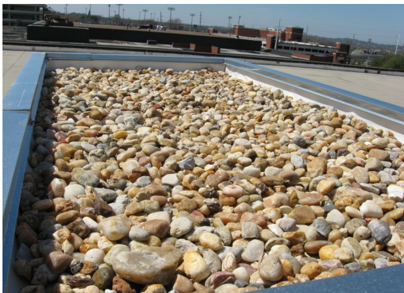
Figure 7. Mini-roof equipped with river rocks.
