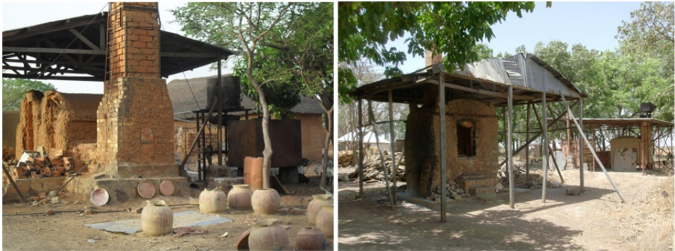
Figure 11. A cross-section of the clay firing facilities (kilns) at Jacaranda and Maraba Pottery Centres
