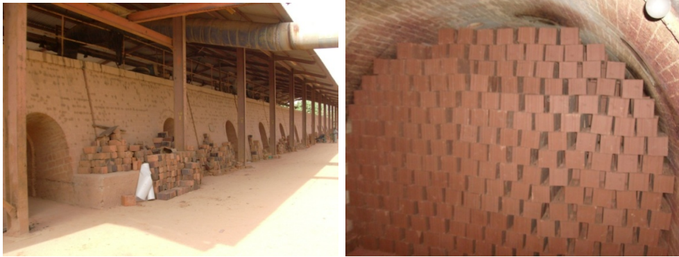
Figure 8. Tunnel kiln and its inner chamber
