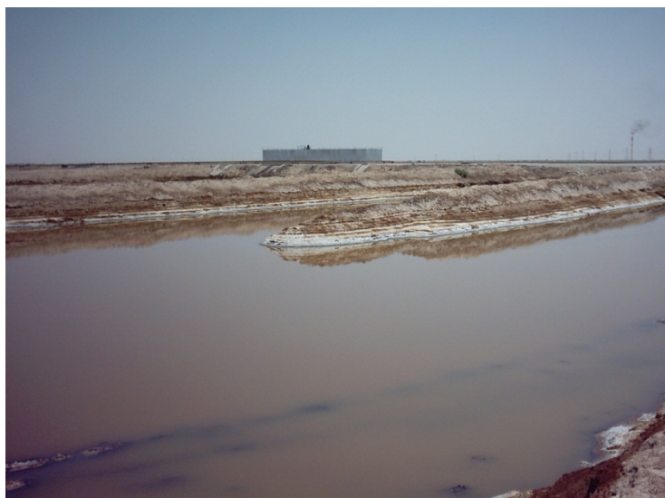
Figure 4. Mud pit condition after drilling operation.
