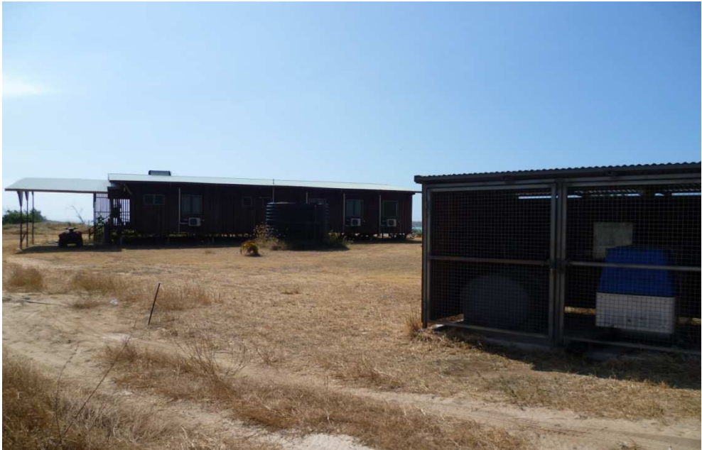
Fig. 7. The Generator Housing in the Foreground and the Dhanaya House
