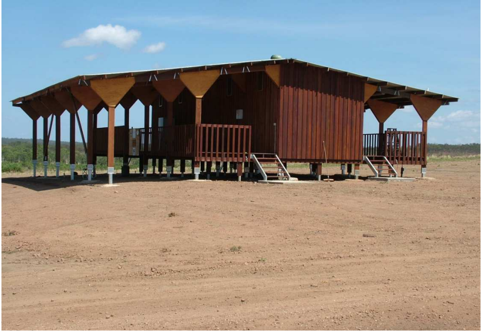
Fig. 5. The Garrathiya Five Room Bunkhouse
