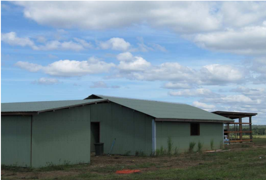
Fig. 3. The Garrathiya Dormitory and Outbuildings during Construction
