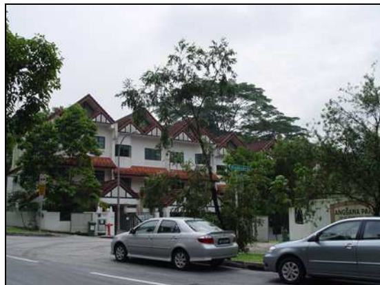
Fig. 2. One of the condominiums just outside the forest
