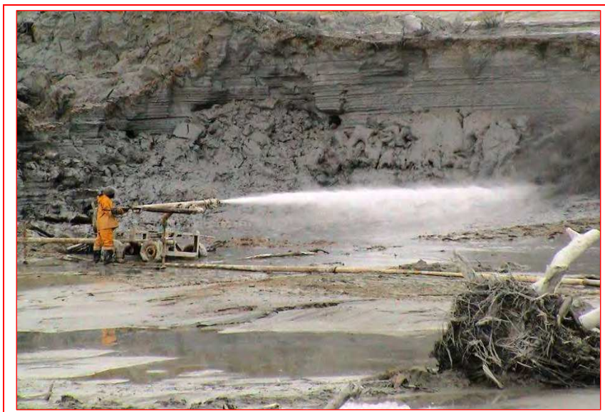
Fig. 2. Monitoring method being used for preparing slimes tailings for reprocessing at Crown Mines.
