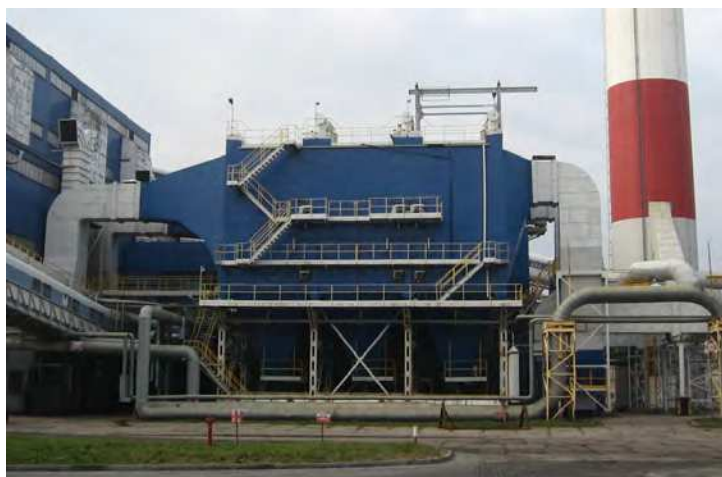
Fig. 1. Electrostatic precipitator in Thermal-Power Station.
