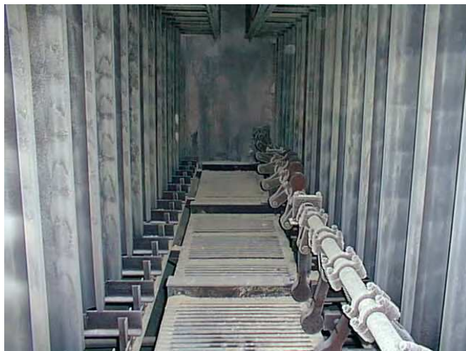
Fig. 2. Inner part of the ESP.
