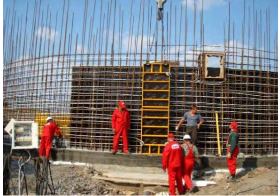
Fig. 11. Building the digester wall for a commercial biogas plant
