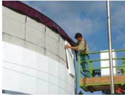
Fig. 17. Installing the insulation (BIOGAS NORD GmbH)
