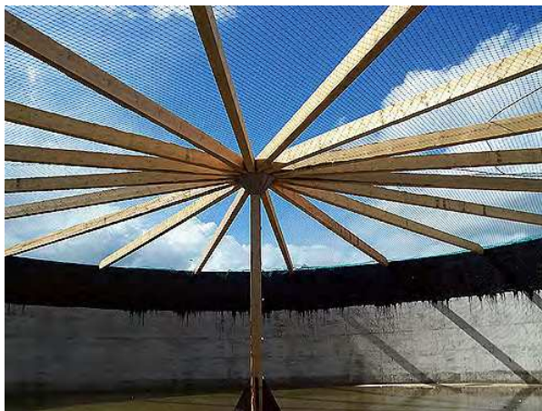
Fig. 14. Wood structure and mesh network that supports the gas holder of digester in a commercial biogas plant (MT-ENERGIE GmbH & Co. KG)
