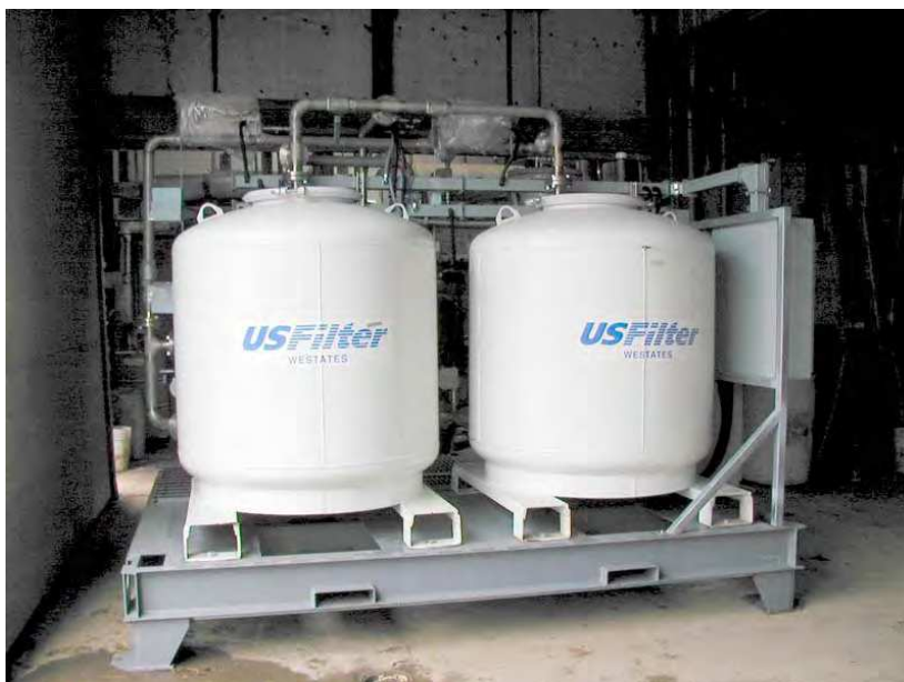
Fig. 19. Activated carbon beds of the GPU (Chandrasekar, 2006)
