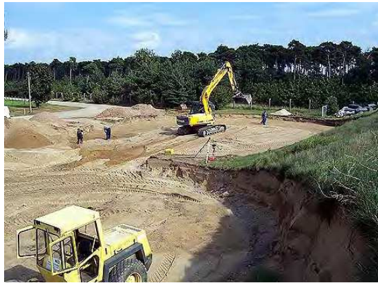
Fig. 7. Excavation works for a commercial biogas plant
