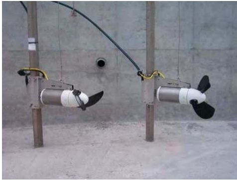
(a) Submersible motor mixing devices
