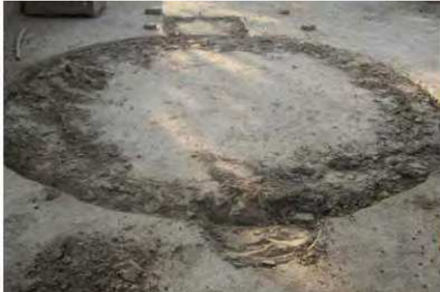
Fig. 5. Marking of dimensions for a biodigester
