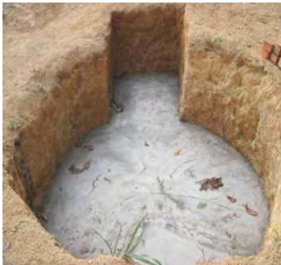
Fig. 10. Concrete bottom of a household unit
