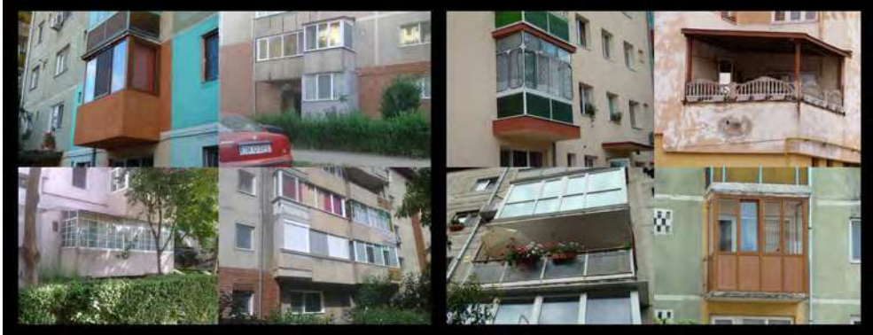
Fig. 27. Modified balconies in the Behaviour Settings of the Blocks of Timișoara City
