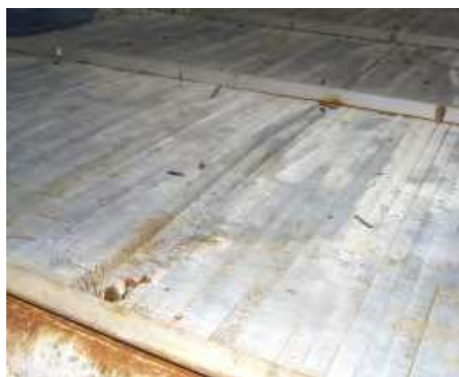
Fig. 2. Buckled tubes of a high performance heat exchanger
